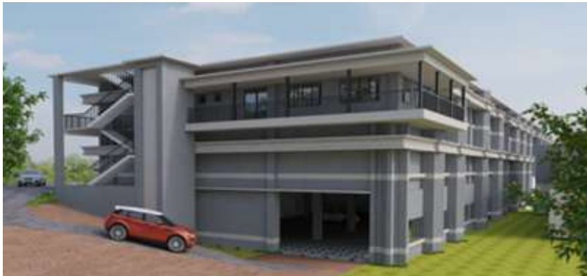
Plinth area of 2448 sq.m Project cost is ₹9.00 Cr
